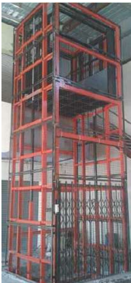
Sky - 132 Hydraulic Goods Lift Double Mast Capacity - 1000/2000/3000kgs Power Pack Operator (Cage Type)
